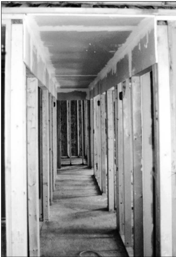
(left) This chase under construction in a ranch style home shows the sealing of the chase with drywall compound. (right) The completed chase.
