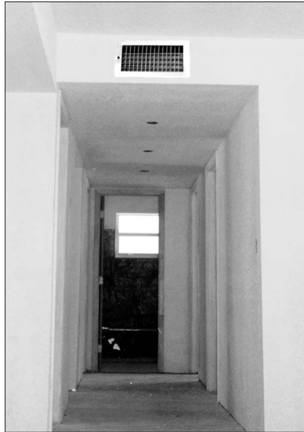
(left) This chase under construction in a ranch style home shows the sealing of the chase with drywall compound. (right) The completed chase.
