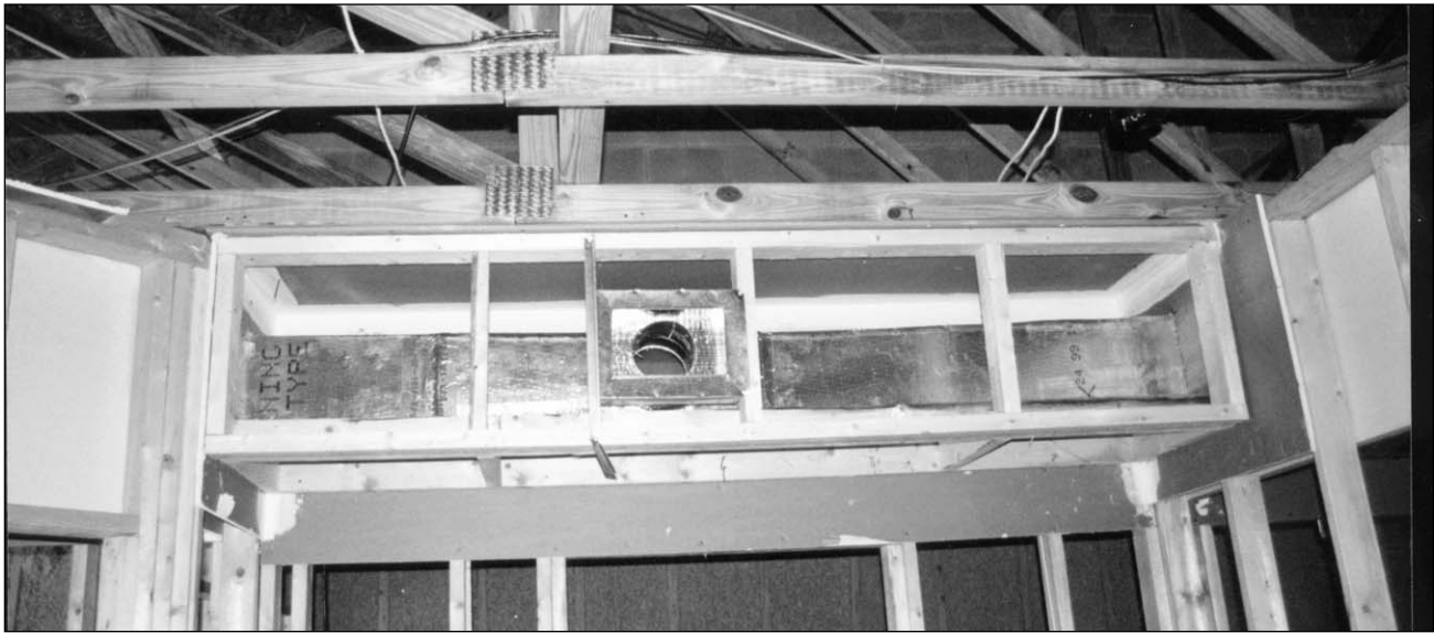
(above) The framer and drywall crew need to take special care in making sure that the chase is properly installed. The site supervisor has to make sure that the integrity of the chase is not compromised. (left) Ken Fonorow points out the spray paint marking the chase location during home construction.
